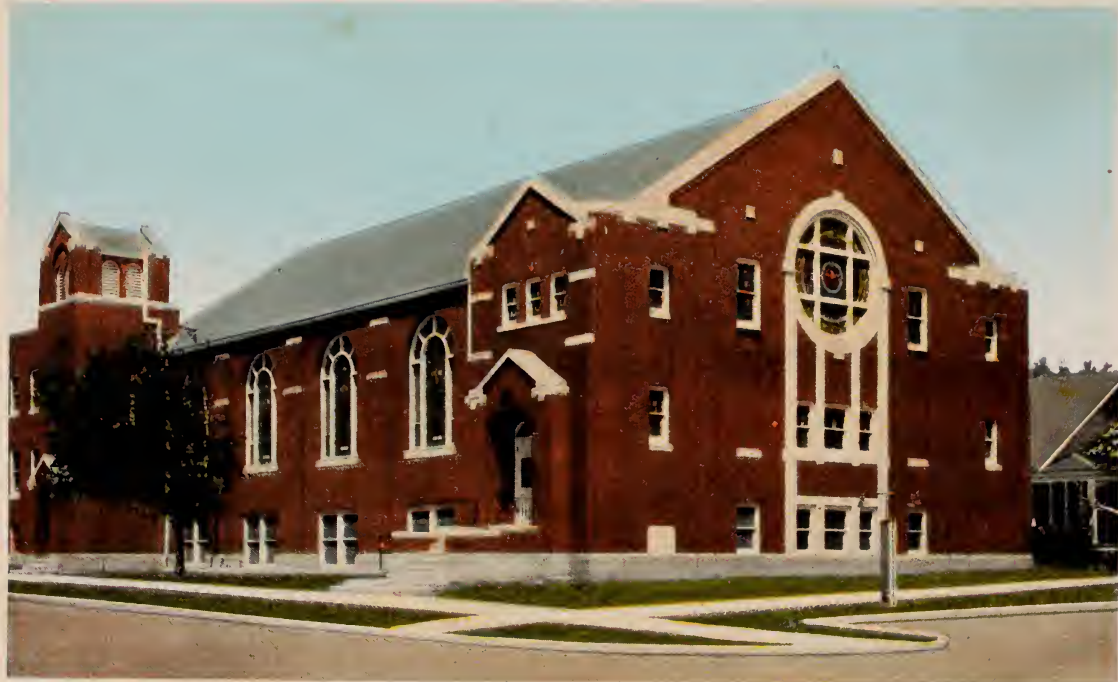
FIRST METHODIST EPISCOPAL CHURCH, CUSHING, OKLA.
